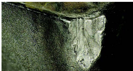
Fracture from welding chipping
